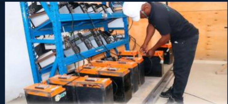
Maintenance Station Sepeda Motor Listrik
